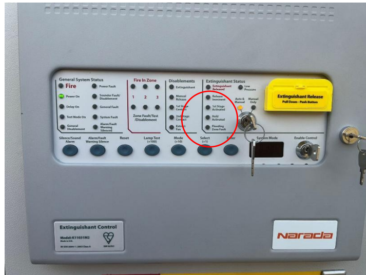
Figure 4-4 FSS Control Panel Auto/Manual Switch (For reference)
